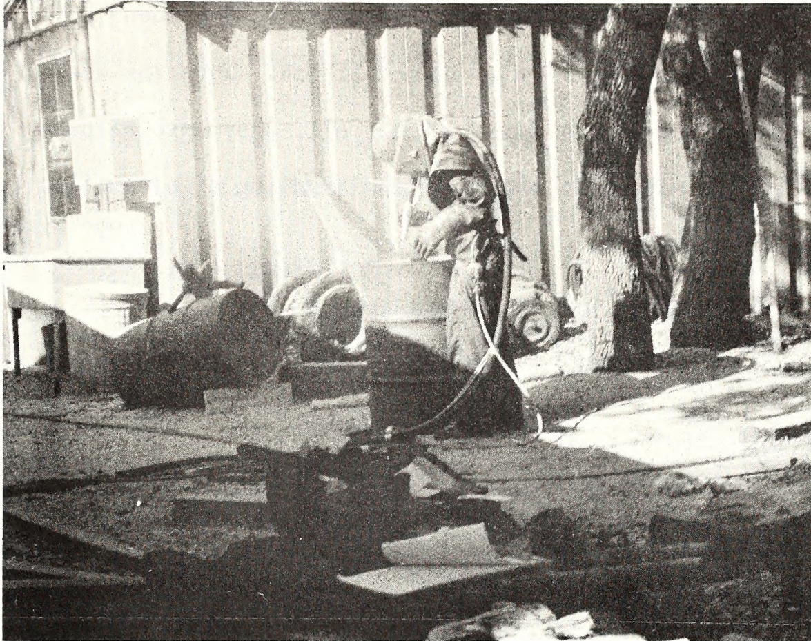
Figure 53. Sandblasting metal carriage parts
